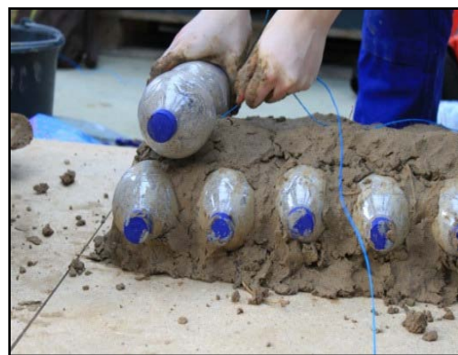
Figure4. Plastic bottles being laid during construction [10]
